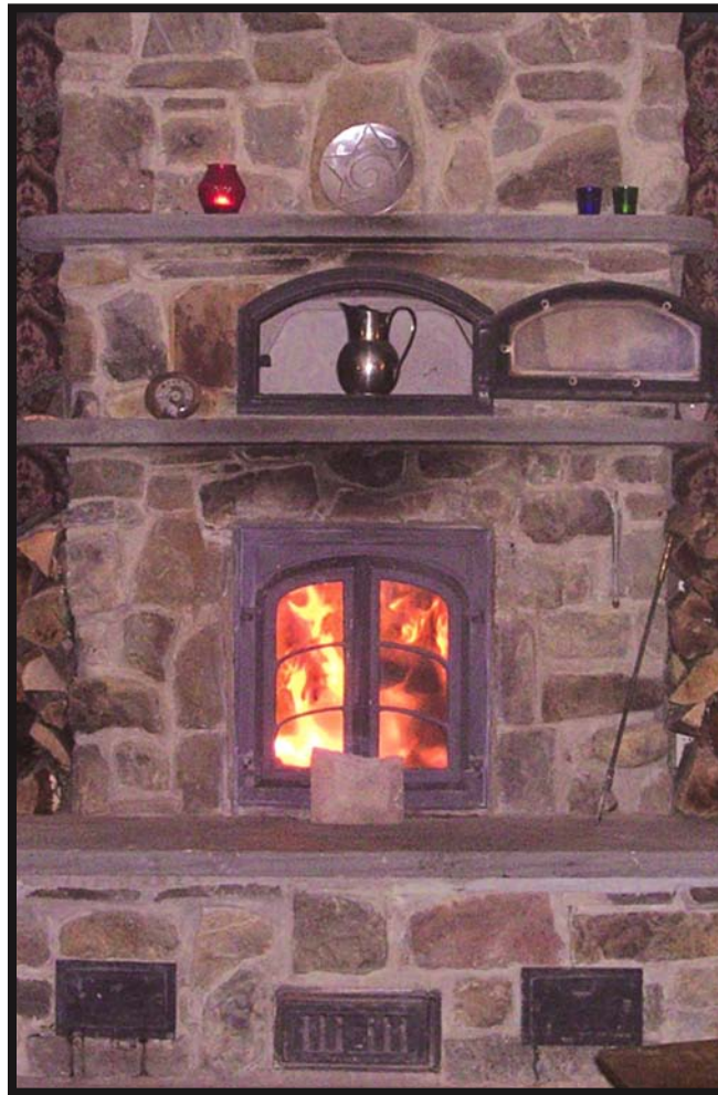
This masonry stove is the focal point of the author's living room and provides soft radiant heat long after the fire is out.
