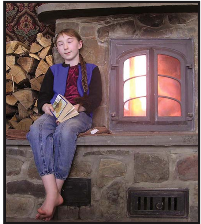
The author's daughter Lexa demonstrates efficient basking behavior, warming herself against the warm (but not hot) thermal mass of the masonry stove.
